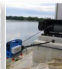
Washington DC Aqueduct Project
